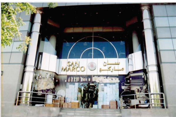
Column and Signages
